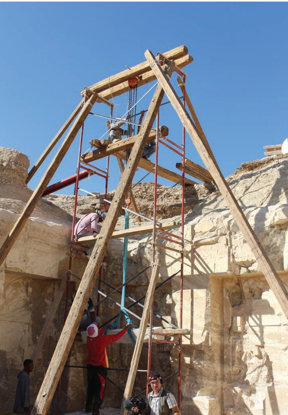
Winch and pulley in the open court
